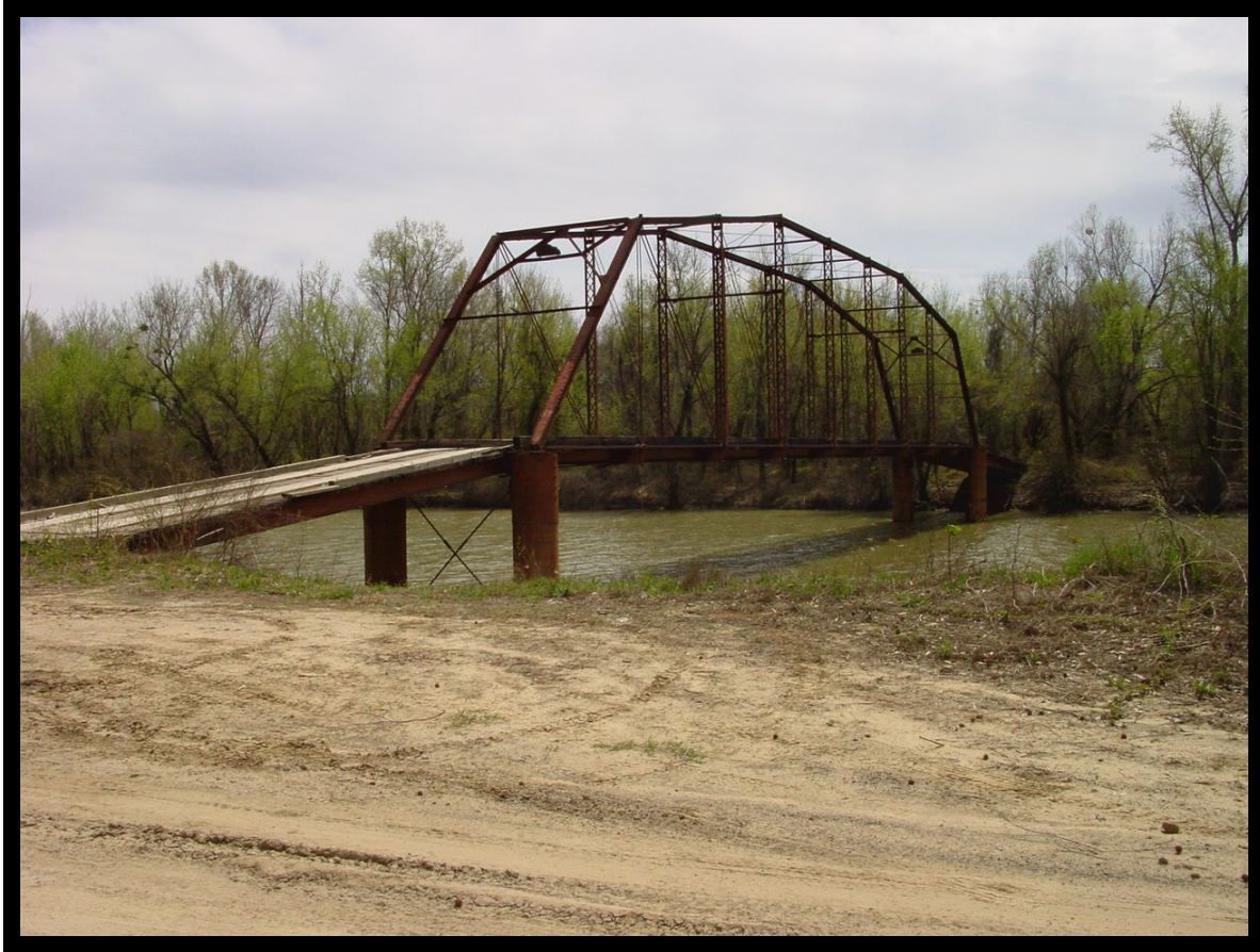
Figure 2. The Ward's Crossing Bridge
