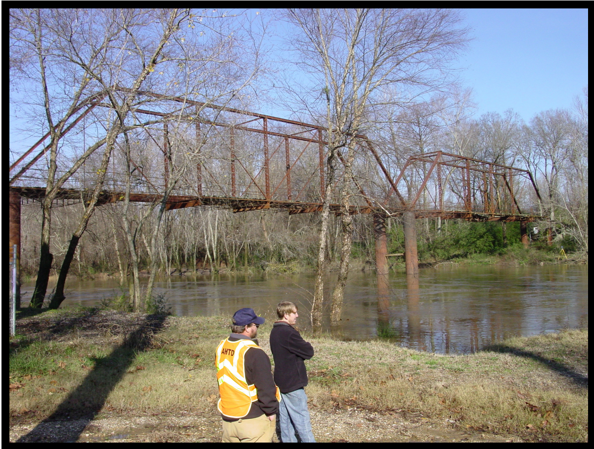
Figure 1. The Old River Bridge
